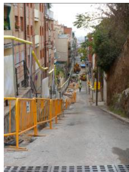
C/Verdi: Vista general
